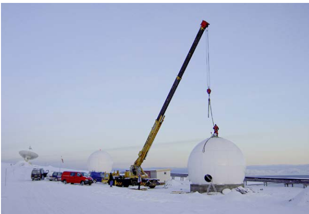
Fig. 4: Installation of the second antenna (NYA-2) in 2005
