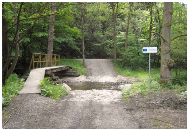
Fig. 3: Part of a new road with a water ford
