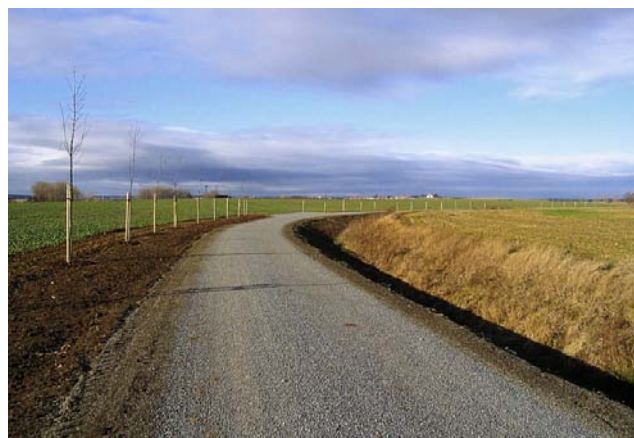
Fig. 2: Newly built dirt road with water ditch and green vegetation planted along it
